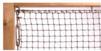
Hogging every mesh to the wire rope ensuring that the net is pulled tight and is square. Attach the other 3 corners using net corner ties. Trim off any surplus net.
