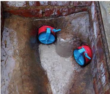
Simple to install the watertight 110 mm non-return valve can help prevent backflow flooding due to floods or sewer blockages. Rats are prevented from entering the property via the drains. Noxious fumes from the sewer system are also unable to escape.
